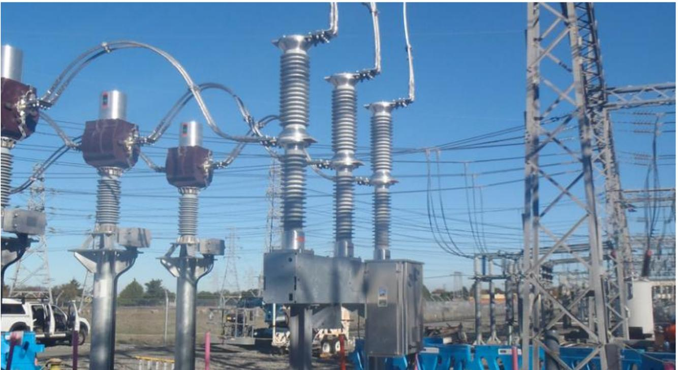
Almost all modern high voltage circuit breakers running at transmission voltage levels employ sulphur hexafluoride ( $\text{SF}_6$ ) as an arc-extinguishing medium for current interruption and for dielectric insulation between the terminals. This is because of the excellent interrupting capabilities of  $\text{SF}_6$ , combined with a high dielectric withstand. However,  $\text{SF}_6$  is a greenhouse gas with high global warming potential.
