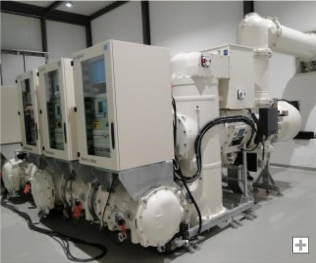
145 kV g3-GIS successfully achieved the high voltage tests at Axpo substation, Etzel, in Switzerland
